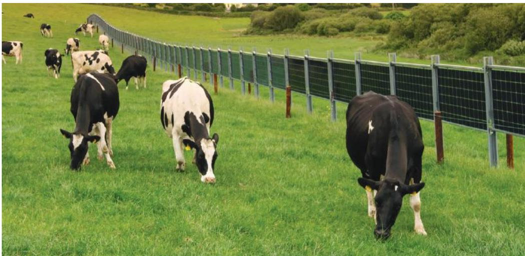
**Figure 6:** Bifacial solar modules fence for livestock enclosure
